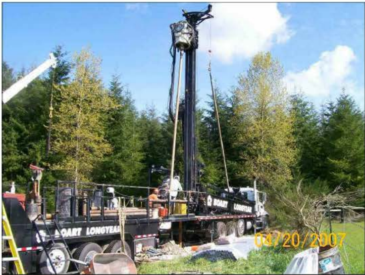
Installing a well at Webb Hill.
